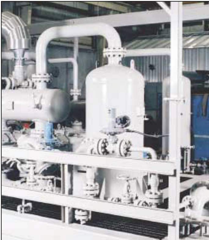
Figure 1. Typical vertical knockout drum
